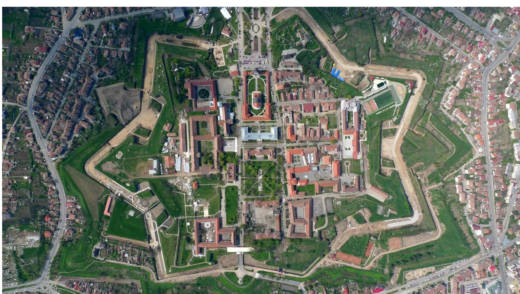
Fig. 1: Aerial view of the Alba Iulia Carolina Fortress.
