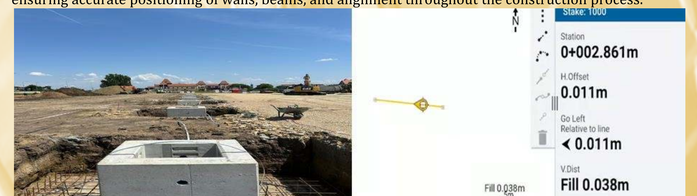
Fig. 6 Axis stakeout using stakeout line method in order to determine the center of the prefabricated structure
